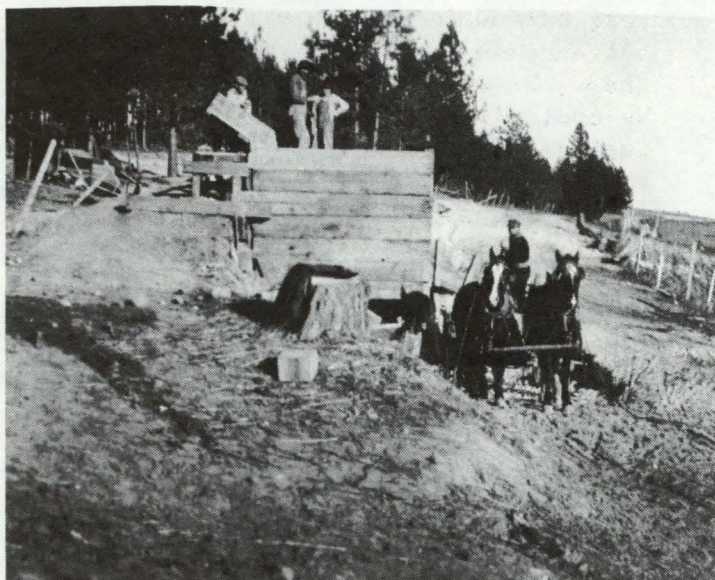
Building the new road near Viola, showing the rock crusher and gravel loaded into wagon.
