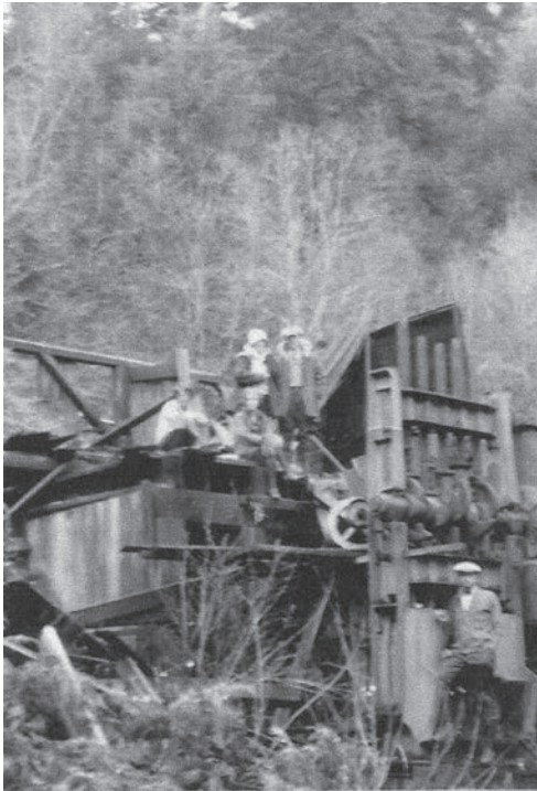
There was an old stamp mill "above cabin" – a good uphill hike of two miles from the Mitchell cabin.
