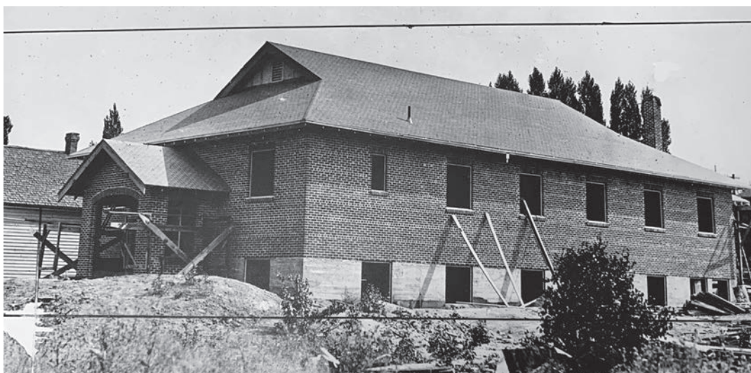
Blue Bucket Inn during construction. 1924. UISPEC PG2_2-93-463
